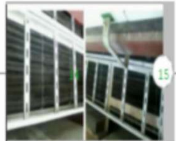
Cable Laying Work ( Control Room )
