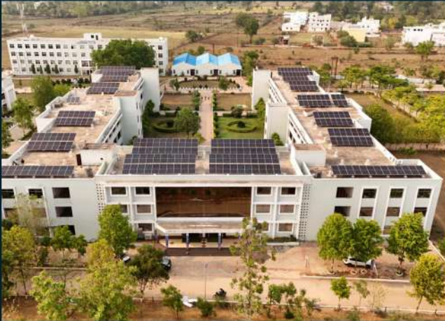
0.25mw ground mounted on grid EPC on Dist. Guna M.P,
