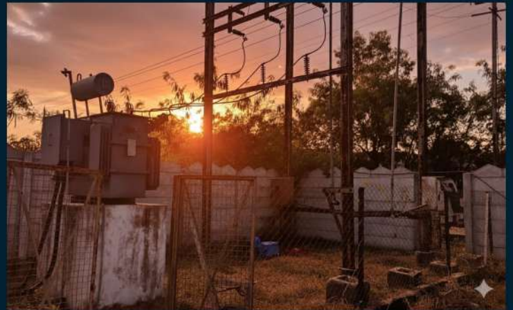
8 mw ground mounted on grid EPC on Chhatarpur M.P.
