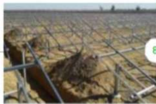
MMS Erection
