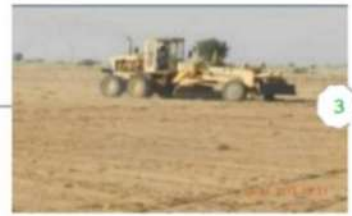
Leveling & Grading
