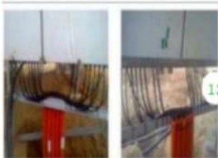
DC Cable Termination (SMB/ SCB Work)
