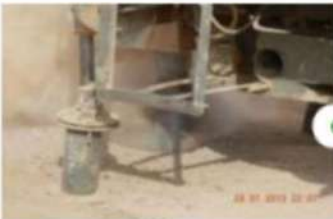
Auguring ( Drilling holes for Foundation )
